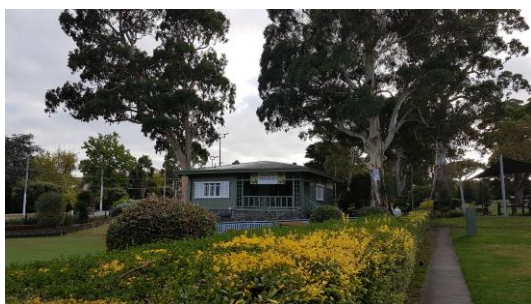
Looking east at Kew Croquet Clubhouse
